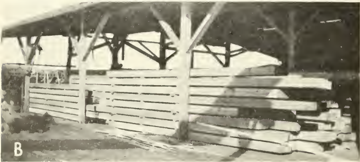
Common practice and good practice in temporary storage: A, Lumber and timbers, in temporary storage, bulk piled unprotected in a loading yard; B, timbers stored temporarily on stickers and under protection from rain and snow, in order to obtain rapid seasoning for the purpose of reducing the likelihood of stain and decay developing during long water shipment
